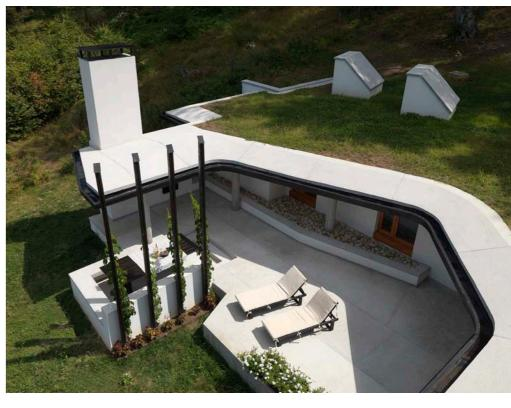
PIR on top, and then 120mm of soil planted with grass on top of that
